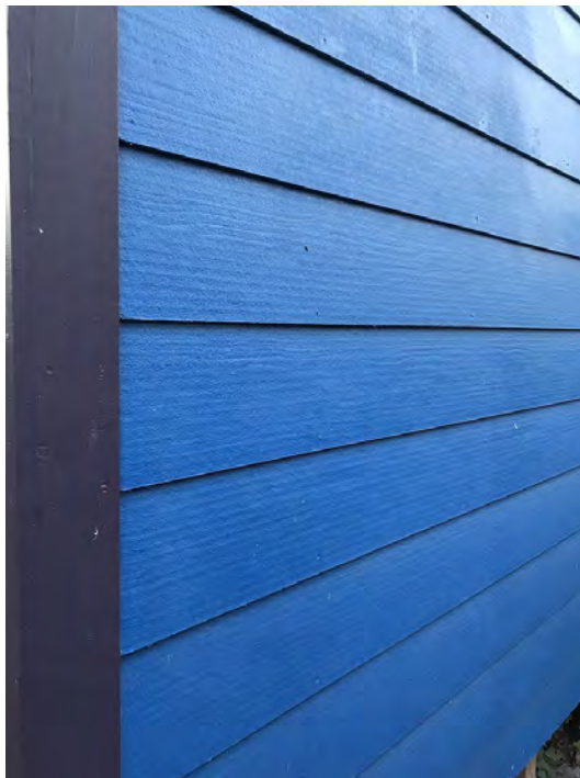
Example of hardboard with flat sides out installation for repair.
